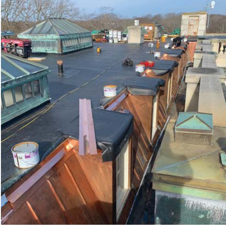
Marble House roof restoration
