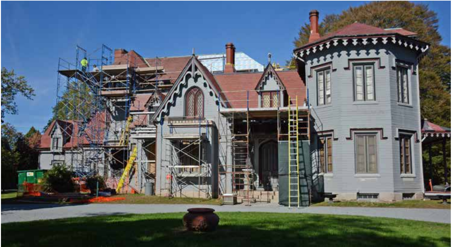
The exterior restoration of Kingscote continued in 2016
