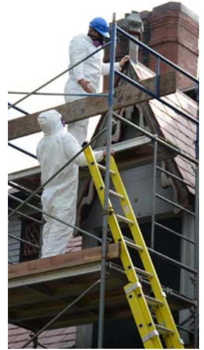
Repairing the details of the Kingscote roof
