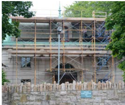
Restoration of The Elms Carriage House
