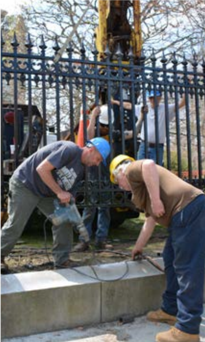
Installing a restored section of The Elms fence
