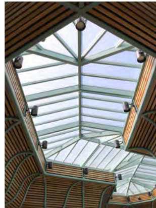
Welcome Center skylight
