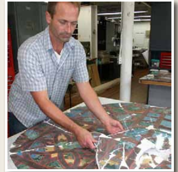
Conservation Assistant John Bartosh re-assembles fragments of the Chateau-sur-Mer stair hall ceiling.
